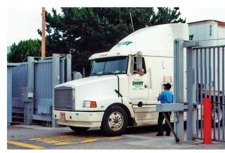
Standard sizes are 108 inches (2.74 m) high and 144 inches (3.65 m) long. Clear openings of up to 33 feet (10 m) may be specified. A non-crash-rated form—the SC3000—is also available.
